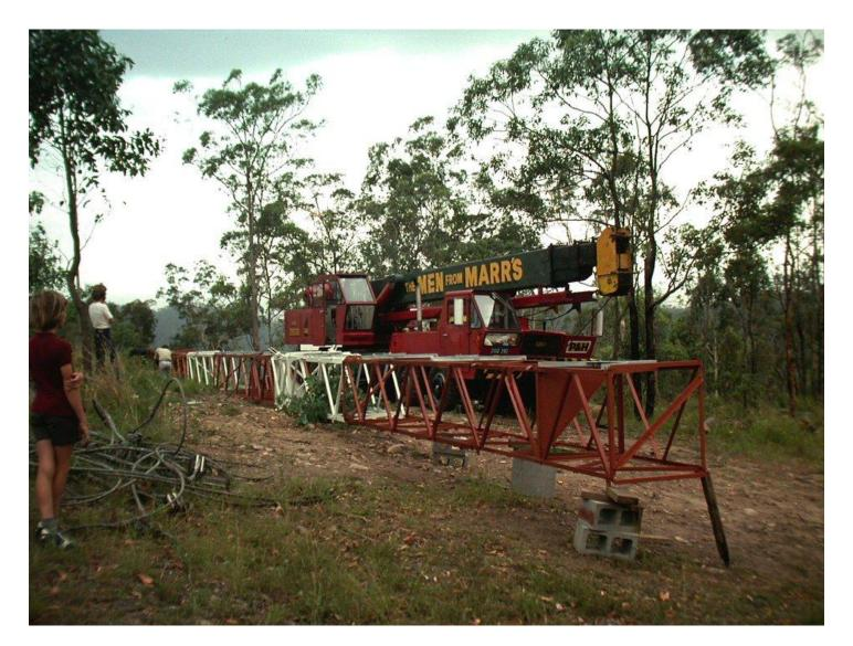
**81.** This tower was relocated from an AM radio transmitter site that had to be removed because of extensions to the Brisbane airport. It was taller than needed, so they removed 30 feet from the top which left a 90-foot mast on which to mount the 4ZZZ antenna. The transmitter was moved to Mount Coot-tha after 4ZZZ was granted a full licence on 30 November 1978. At the same time, the frequency was changed from 105.7 MHz to 102.1 Mhz (a government requirement).
