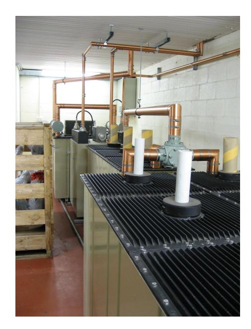
**196.** Downstairs at Broadcasting Park, Mount Coot-tha. The combiner system that joins the five station's signals into the one antenna. Photo: © Gavin Unsworth 2007.
