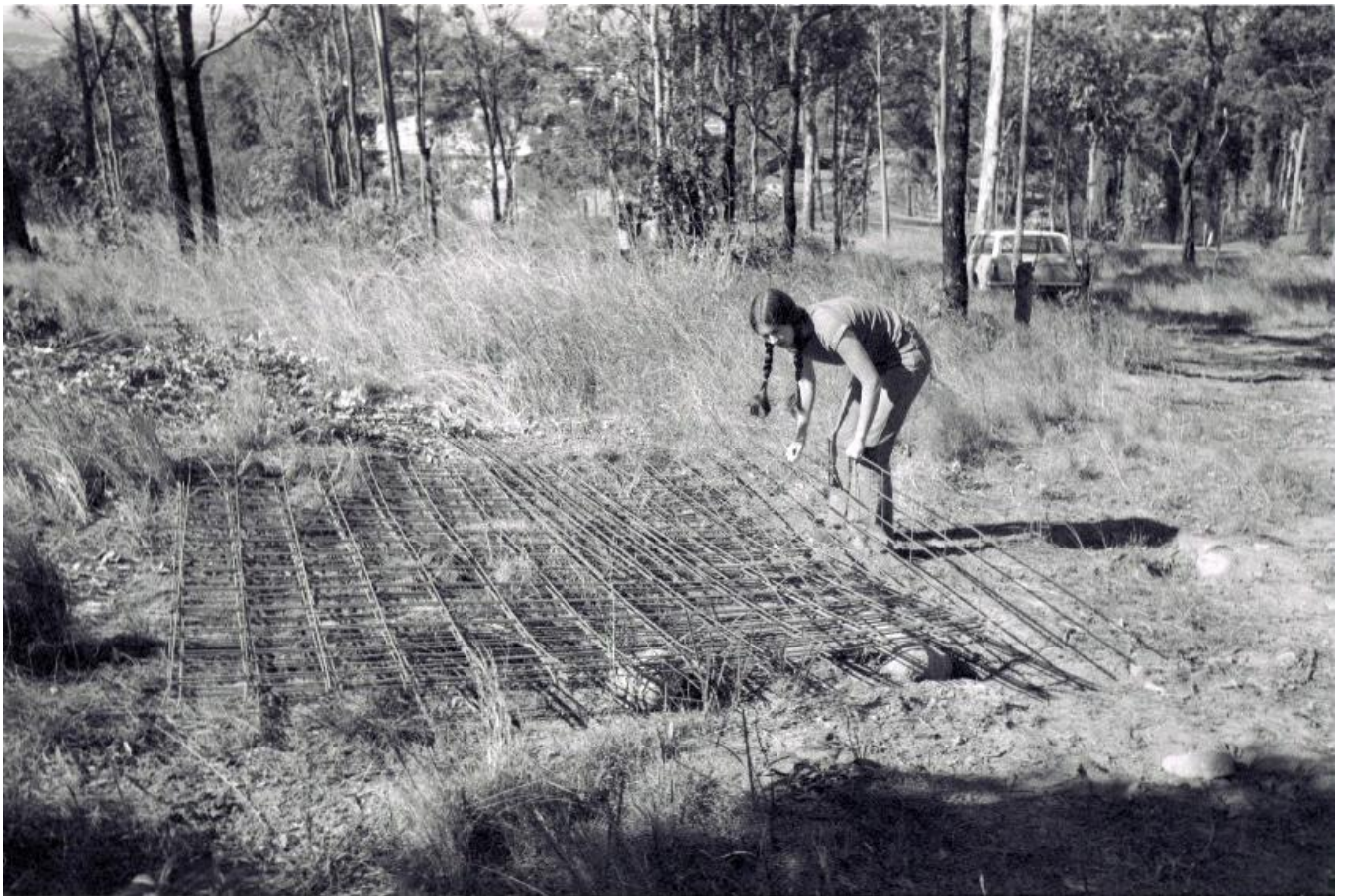
13. Laying steel mesh. (Photograph: © Allan Martin 1977)
