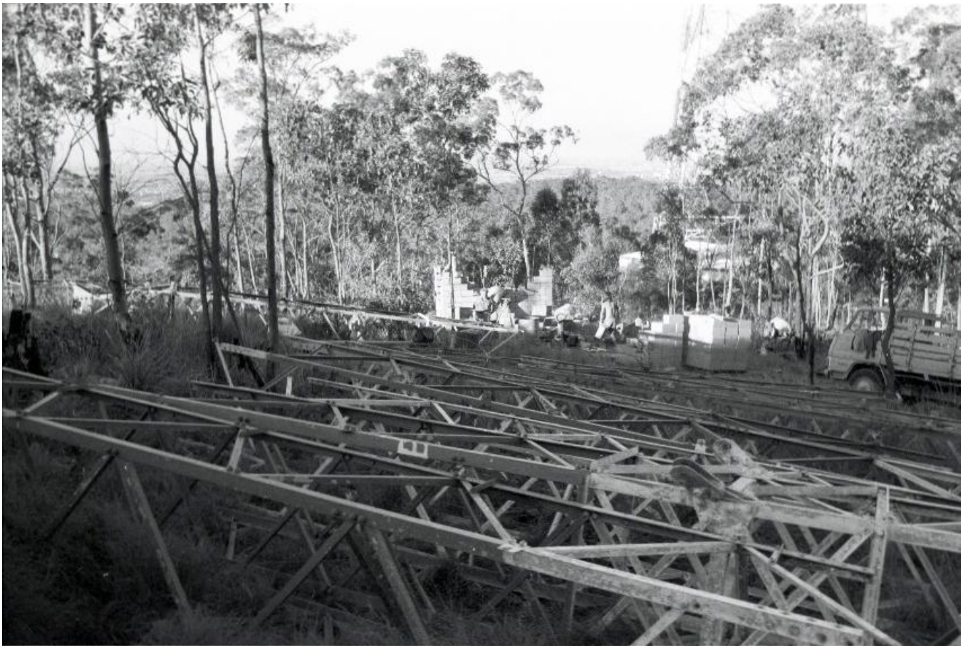
14. Sections of the mast. (Photograph: © Allan Martin 1977)
