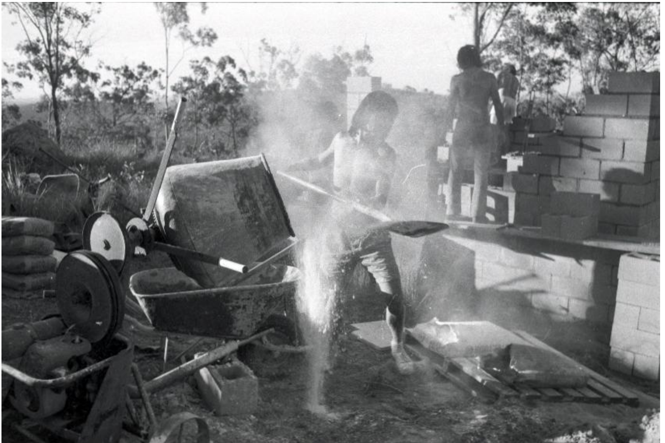
06. Mixing concrete. (Photograph: © Allan Martin 1977)
